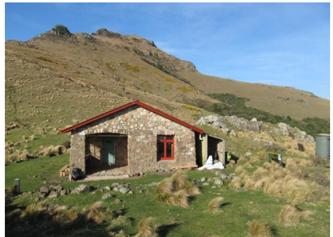
Packhorse Hut 2015, Mt Bradley in the background
